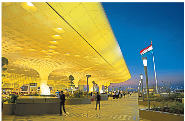
The housing association alleged that MIAL had illegally initiated demolition of 19 vacant buildings at Kalina Air India colony. MINT
