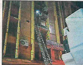
The fire is said to have been caused by a short circuit in an air conditioner. SOURCED
